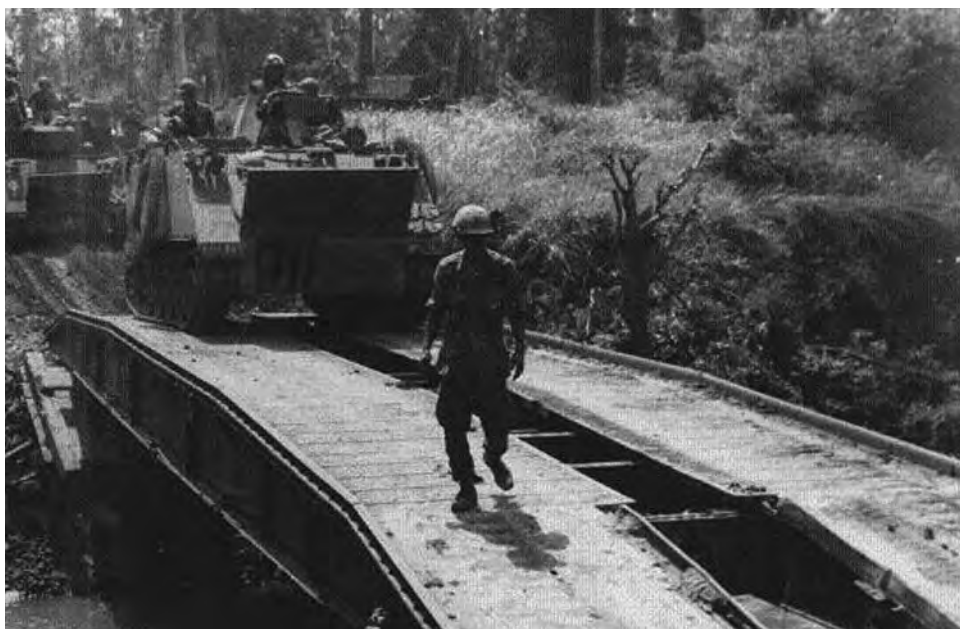
During Operation SHENANDOAH, the 1st Engineer Battalion supported the movement of the division's armored personnel carriers by erecting tactical bridging such as this armored vehicle launched bridge.
